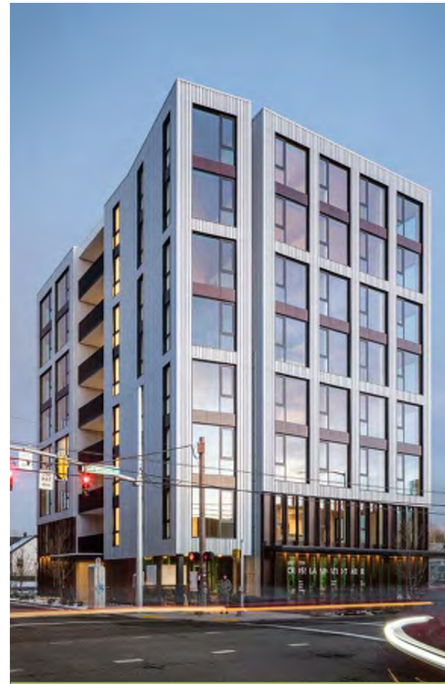
Carbon12 Portland, Oregon | Eight stories of mass timber Kaiser Group and Path Architecture Munzing Structural Engineering
