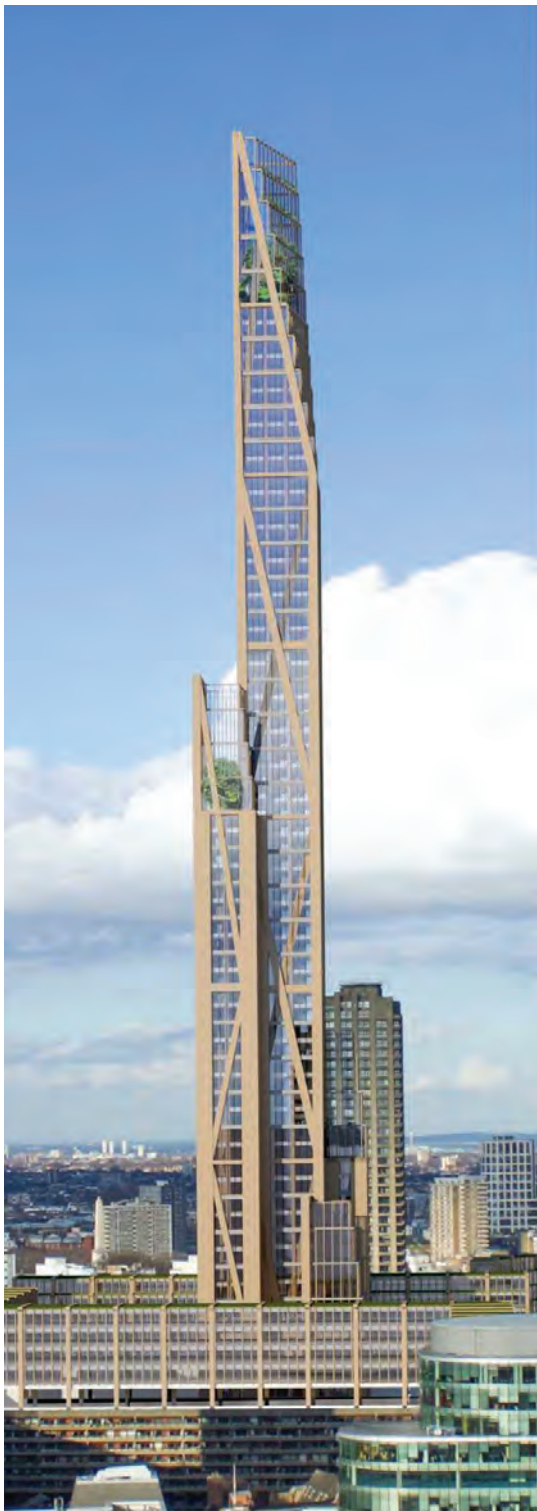
OAKWOOD TOWER - LONDON
