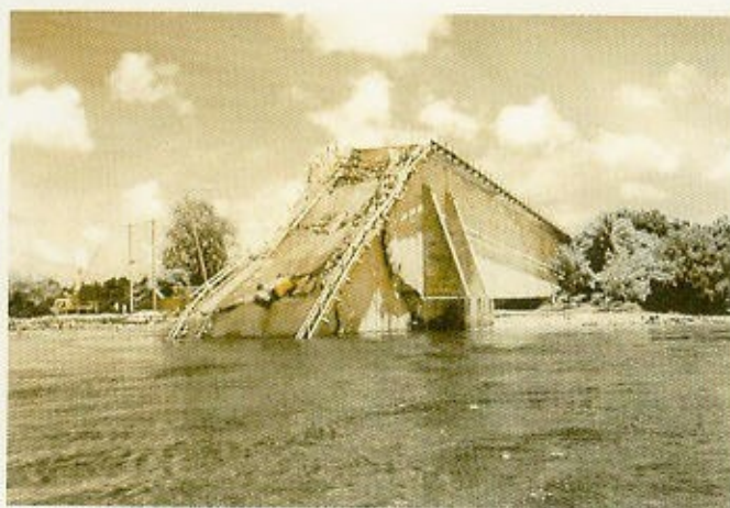
(b) Koror-Babeldaob Box Girder in Republic of Palau, 1996.
