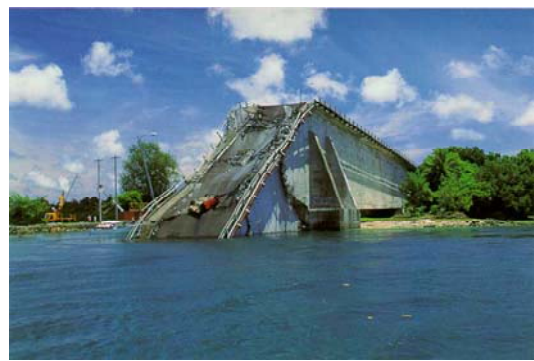
Fig. 10 Examples of Catastrophic Failures of Concrete Structures. (a) Sleipner Oil Platform, 1991; (b) Koror-Babeldaob Box Girder in Republic of Palau, 1996.
