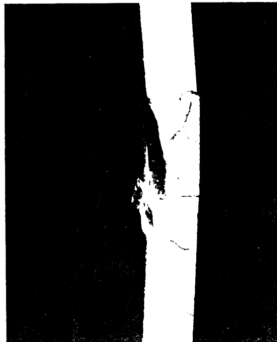
Fig. 2 Typical break of the column.
