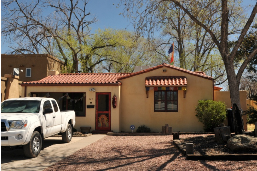
Figure III-1 - West side of the 324 Wellesley House
