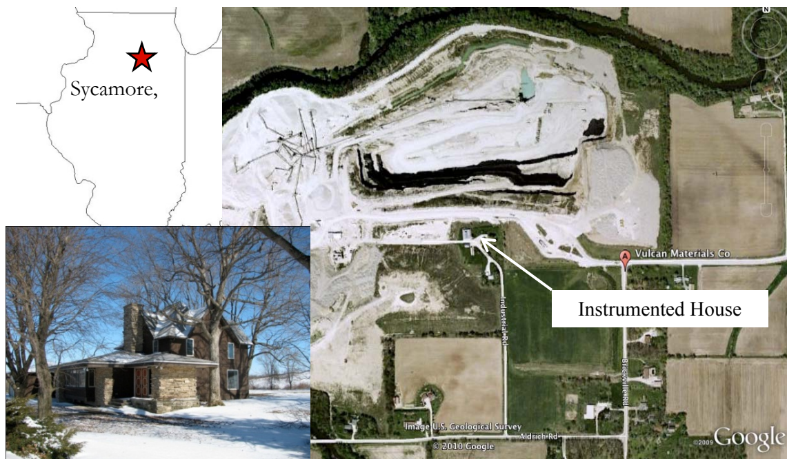
Figure II-1 - Overall view of Vulcan Materials, CO. Sycamore Quarry and photograph and location of the instrumented house
