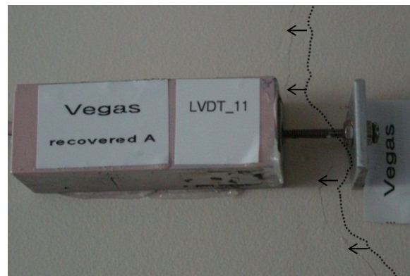
Figure II-3 - Overall views of the wall-mounted crack sensors
