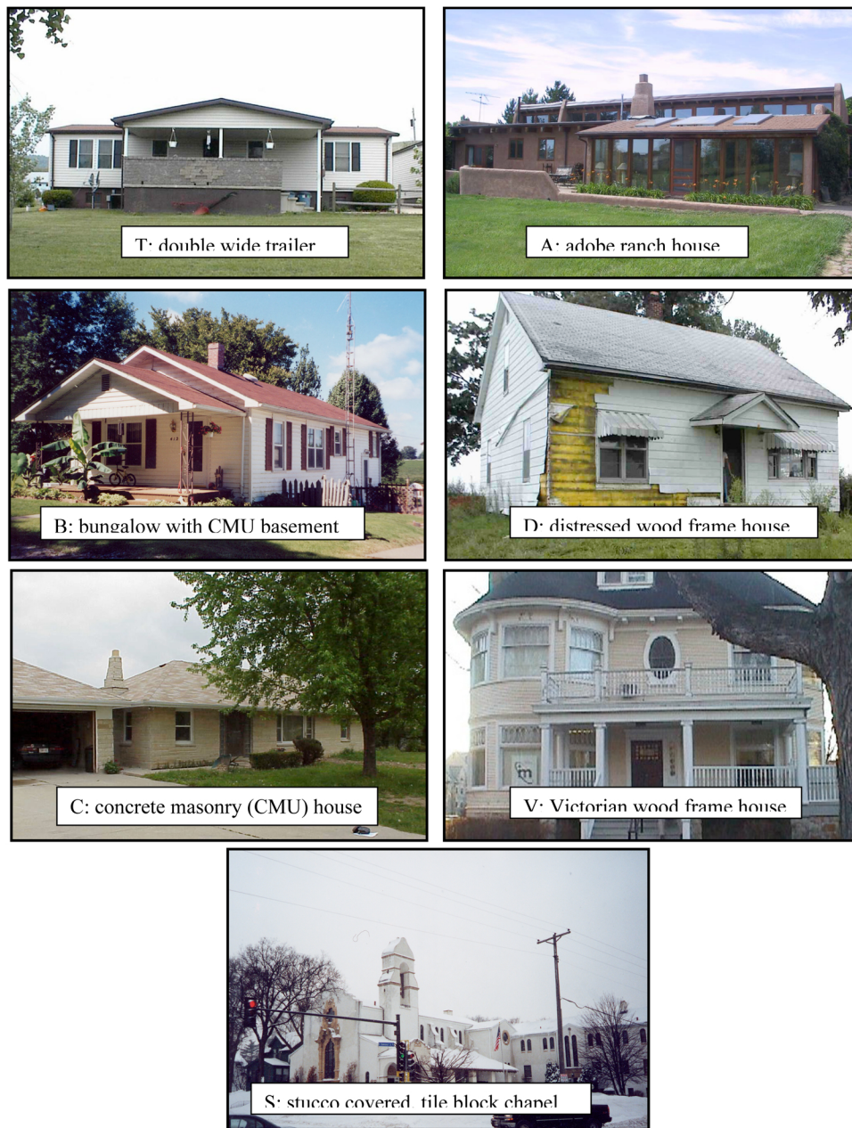
Fig. 3. Seven structures monitored for crack response to long term and transient effects clockwise from top left: T , A , D , V , S , C , and B
