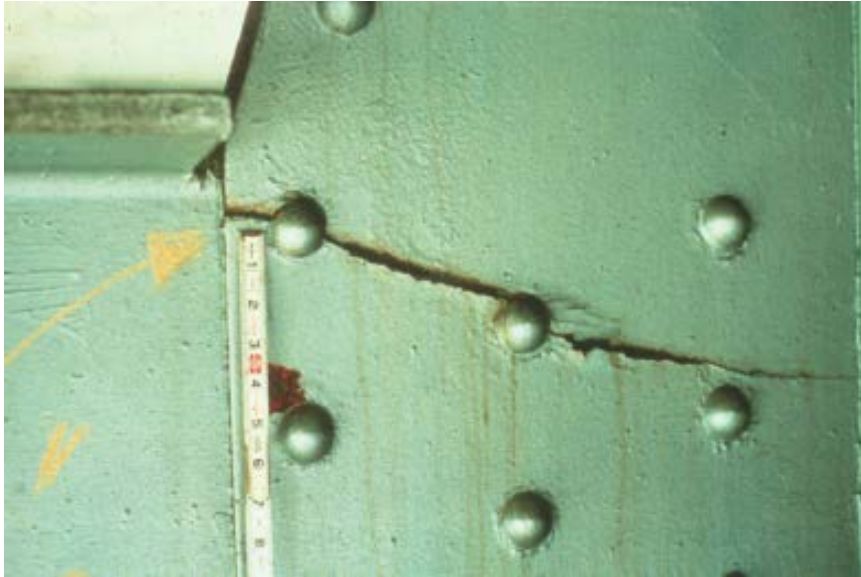
Figure B-1: Fatigue crack at coped top flange of riveted connection, after United States Department of Transportation: Federal Highway Administration (2006)
