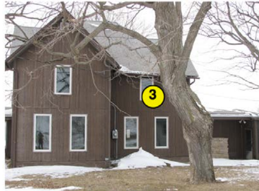
Figure D-6. Exterior view of east wall of instrument test house, showing where Node 3 is inside.
