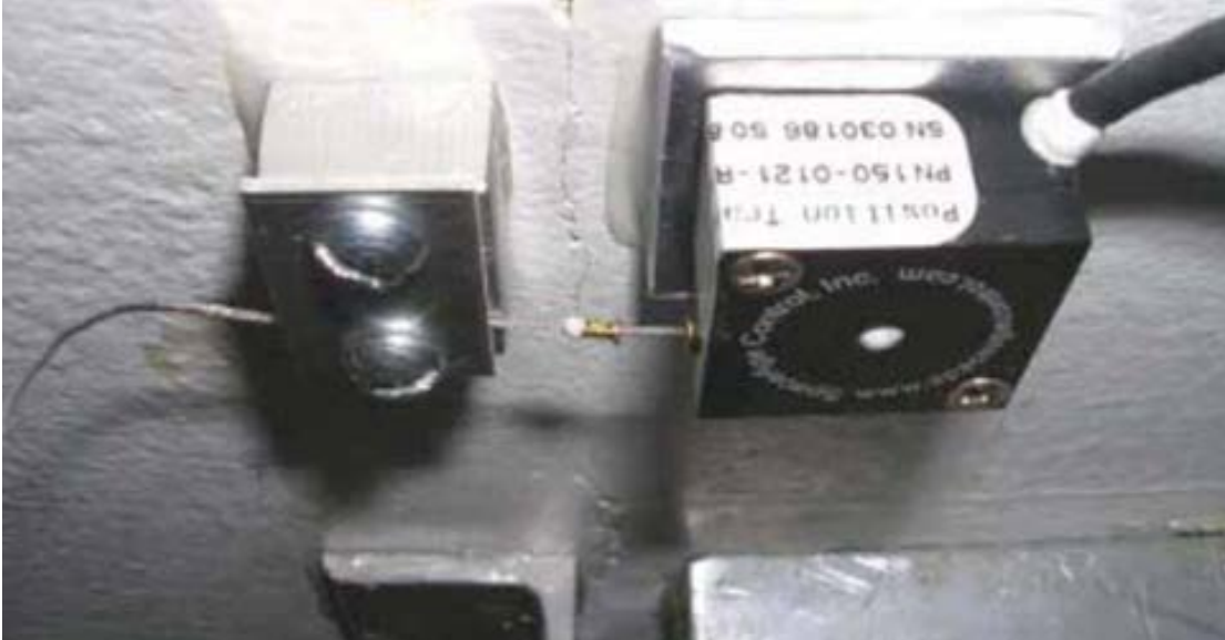
Figure D-17. Details of the potentiometric proximity sensor spanning the ceiling crack.
