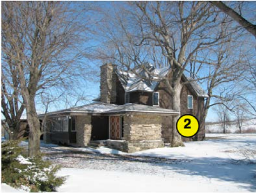
Figure D-5. Exterior view of southwest corner of instrumented test house, showing where Node 2 is inside.
