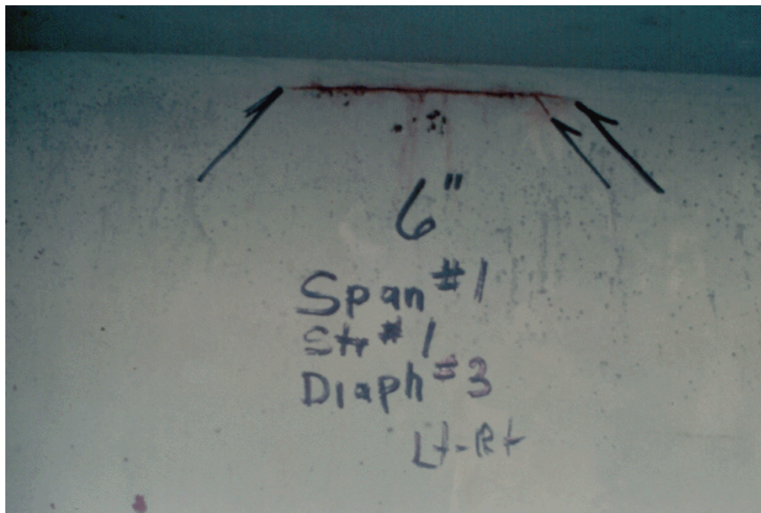
Figure B-1: Fatigue crack at coped top flange of riveted connection, after United States Department of Transportation: Federal Highway Administration (2006)
