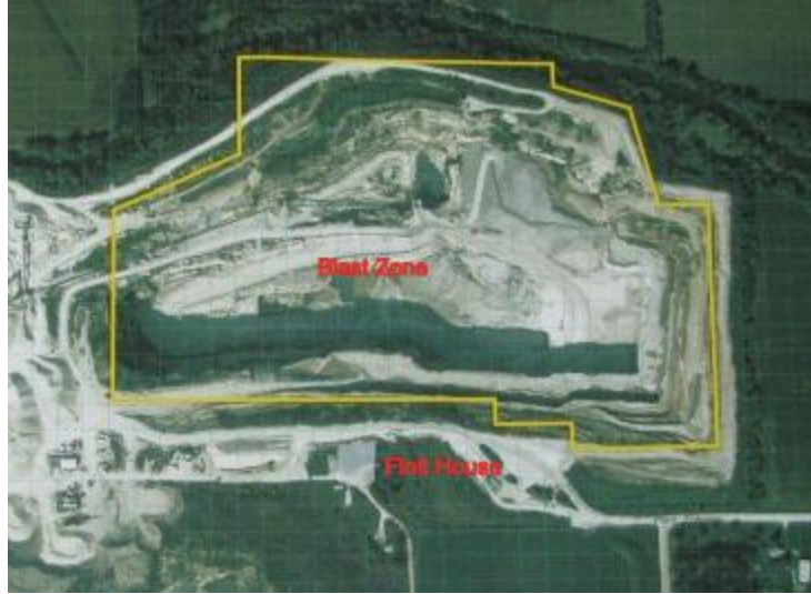
Figure 1: Aerial View of Site with Annotations
