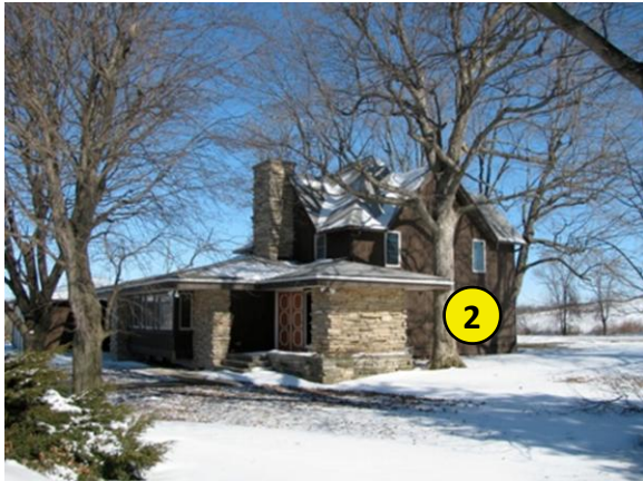
Figure 2.2 - Exterior view of southwest corner of instrumented Floit House, showing where Node 2 is inside.
