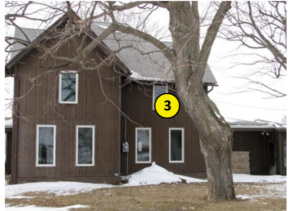
Figure 2.3 - Exterior view of east wall of instrumented Floit House, showing where Node 3 is inside.
