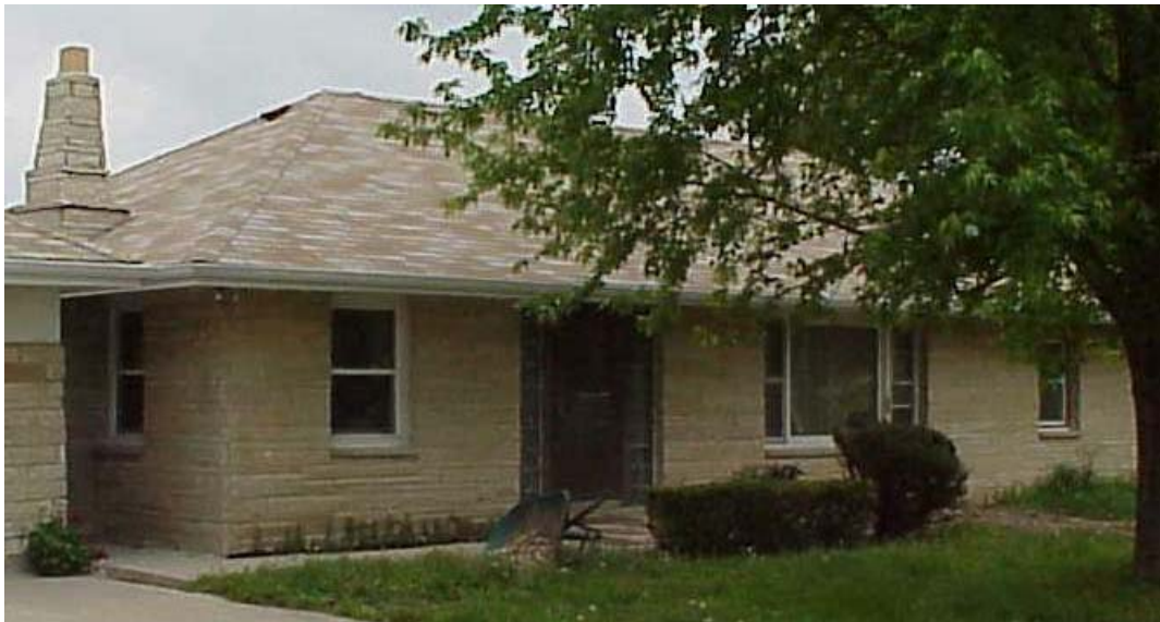
Figure 3.1 Test House Two front view
