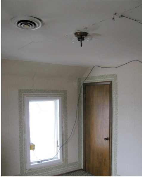
← b - Upstairs bedroom ceiling showing the location of the crack and the transducer
