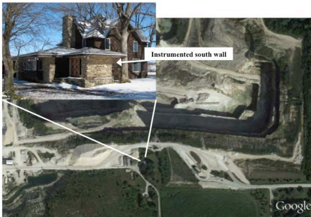
Figure 1. Instrumented house located just south of the quarry. Response of cracks in south wall (indicated by white arrow) under observation at time of the appearance of new crack. Map data © 2013 Google, USDA Farm Service Agency.
