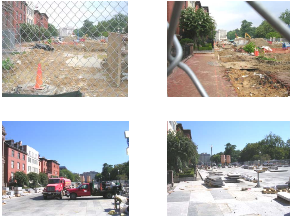
Figure 2-2: Views of street a) during (upper) and b) after (lower) reconstruction.
