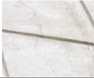
exterior stucco crack 1
