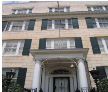
Figure 2-1: Front view of the façade of the instrumented house.
