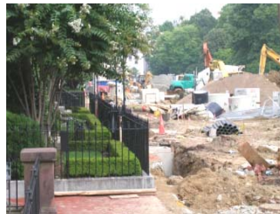
Figure 2-3: Trenching activities within two meters of the structure.
